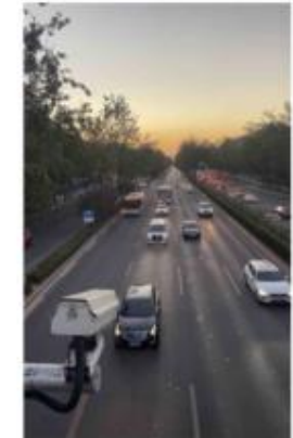
Install a data acquisition system in field
